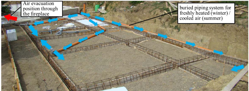
Fig. 4 Pipe system for natural ventilation
